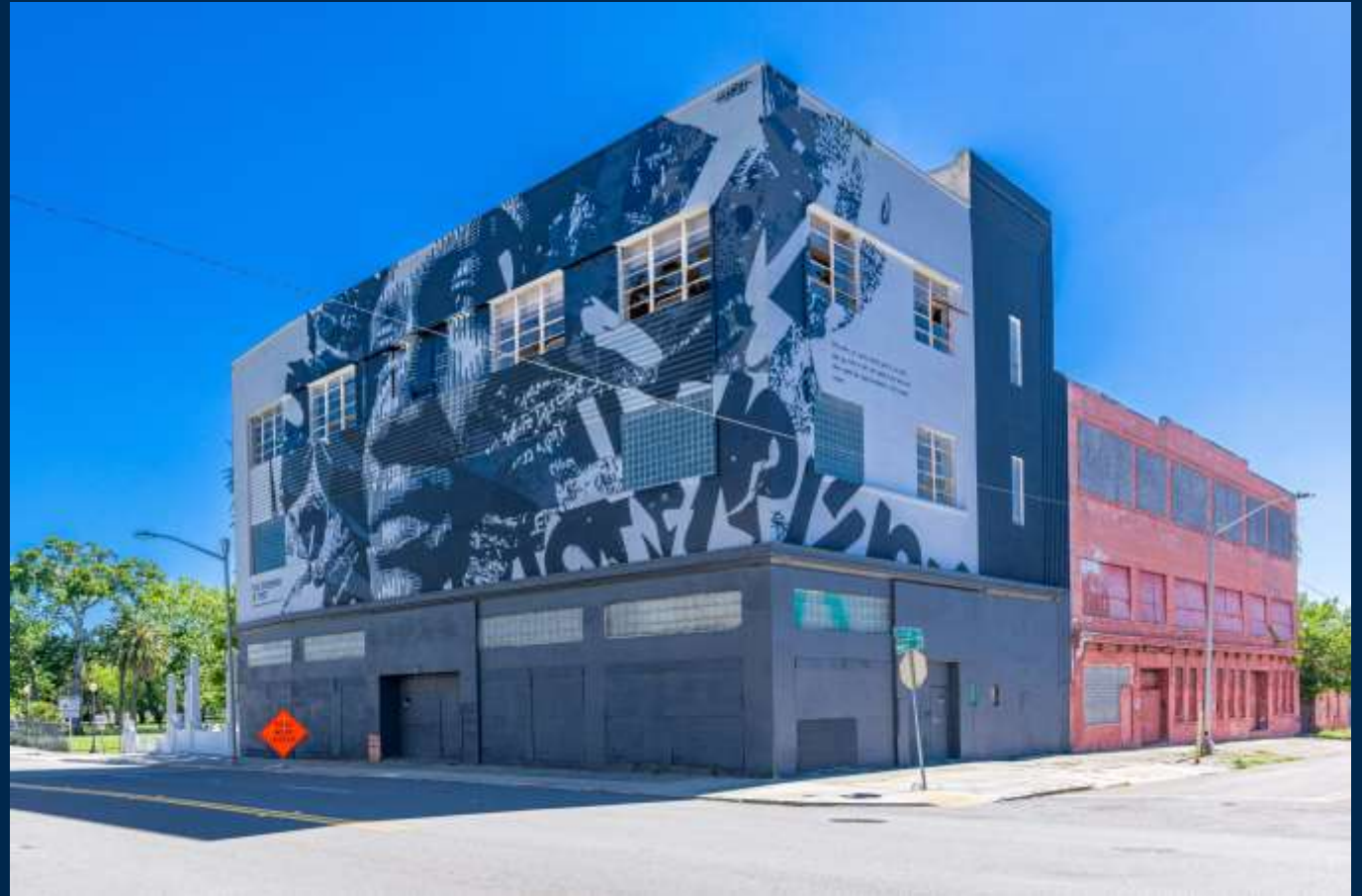
Photo by Mark Krancer, Kram Kran Photo
