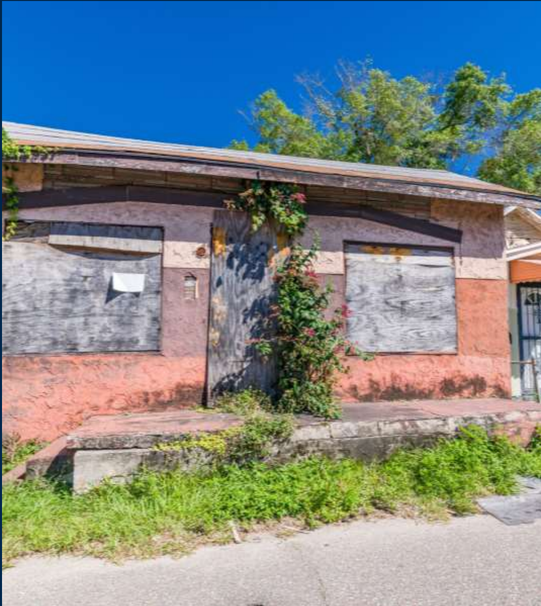
Photo by Mark Krancer, Kram Kran Photo
