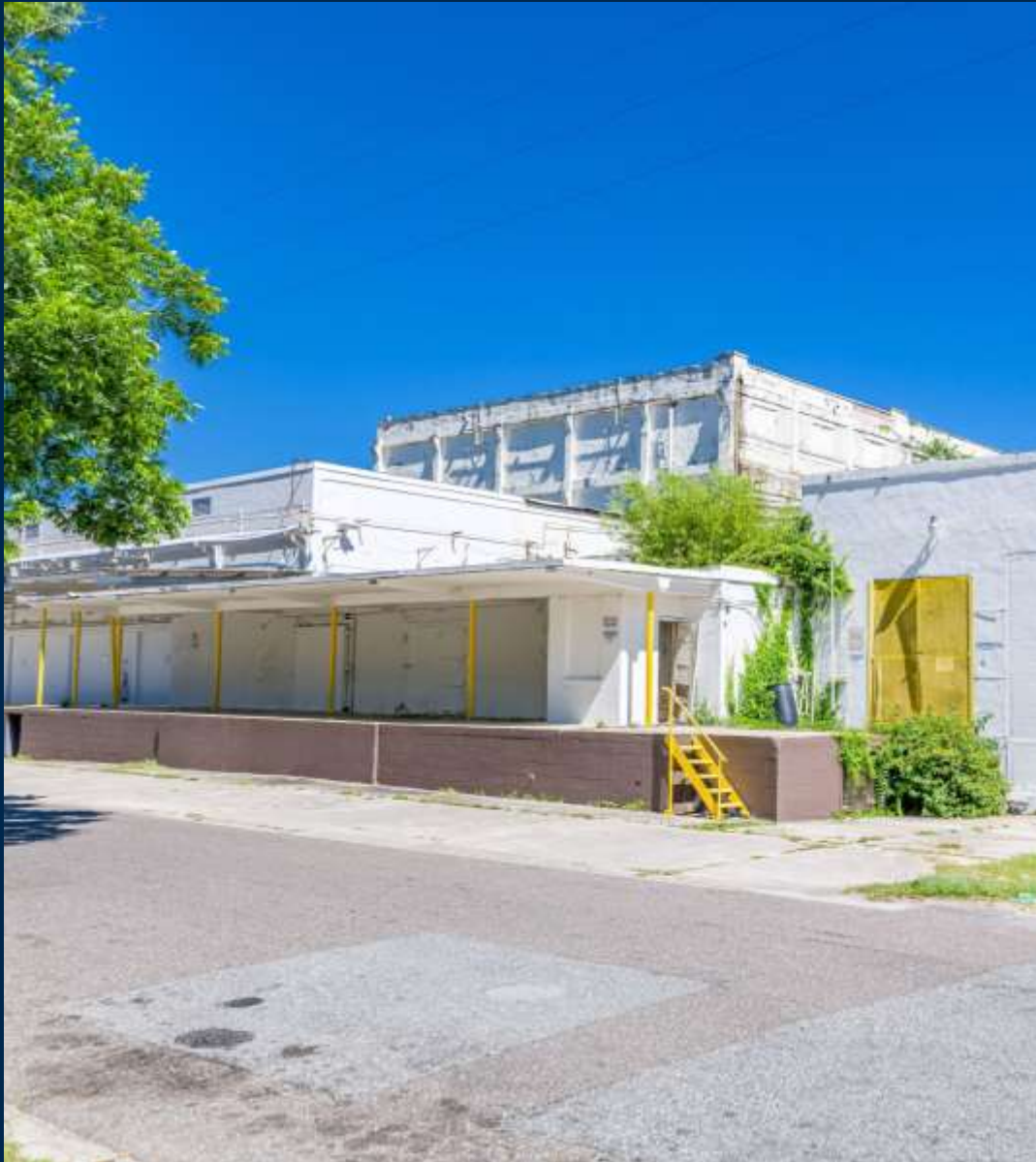
Photo by Mark Krancer, Kram Kran Photo
